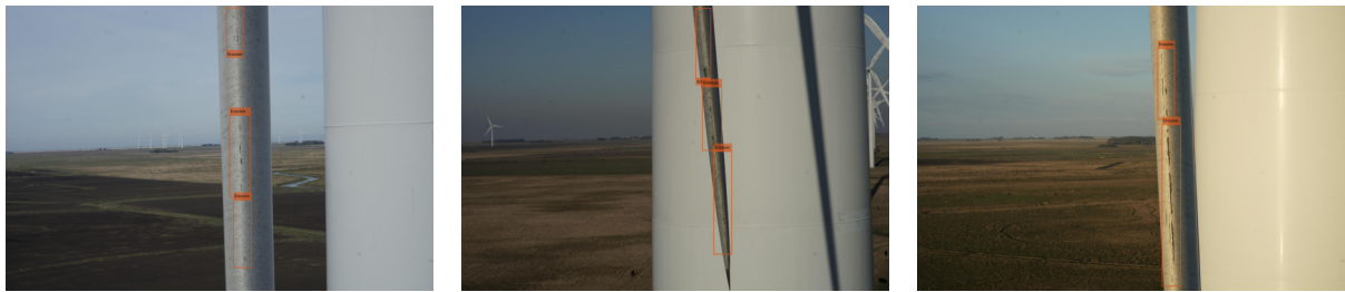
Figure D.1: Examples of Erosion
