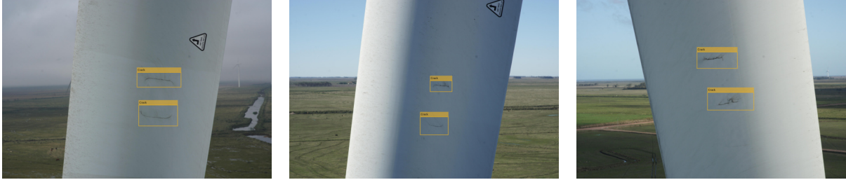
Figure D.3: Examples of cracks
