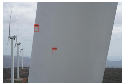
(b) Small peeling of the gel coat
