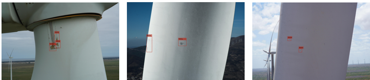
Figure D.2: Examples of peeling
